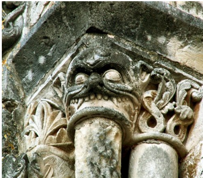
Detail of doorway, Civray (Vienne) click for another photo
