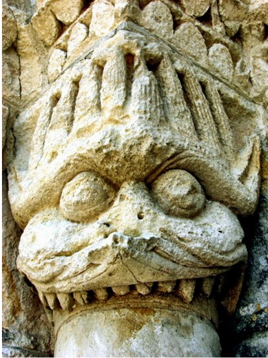
Detail of doorway, Chadénac (Charente-Maritime)
